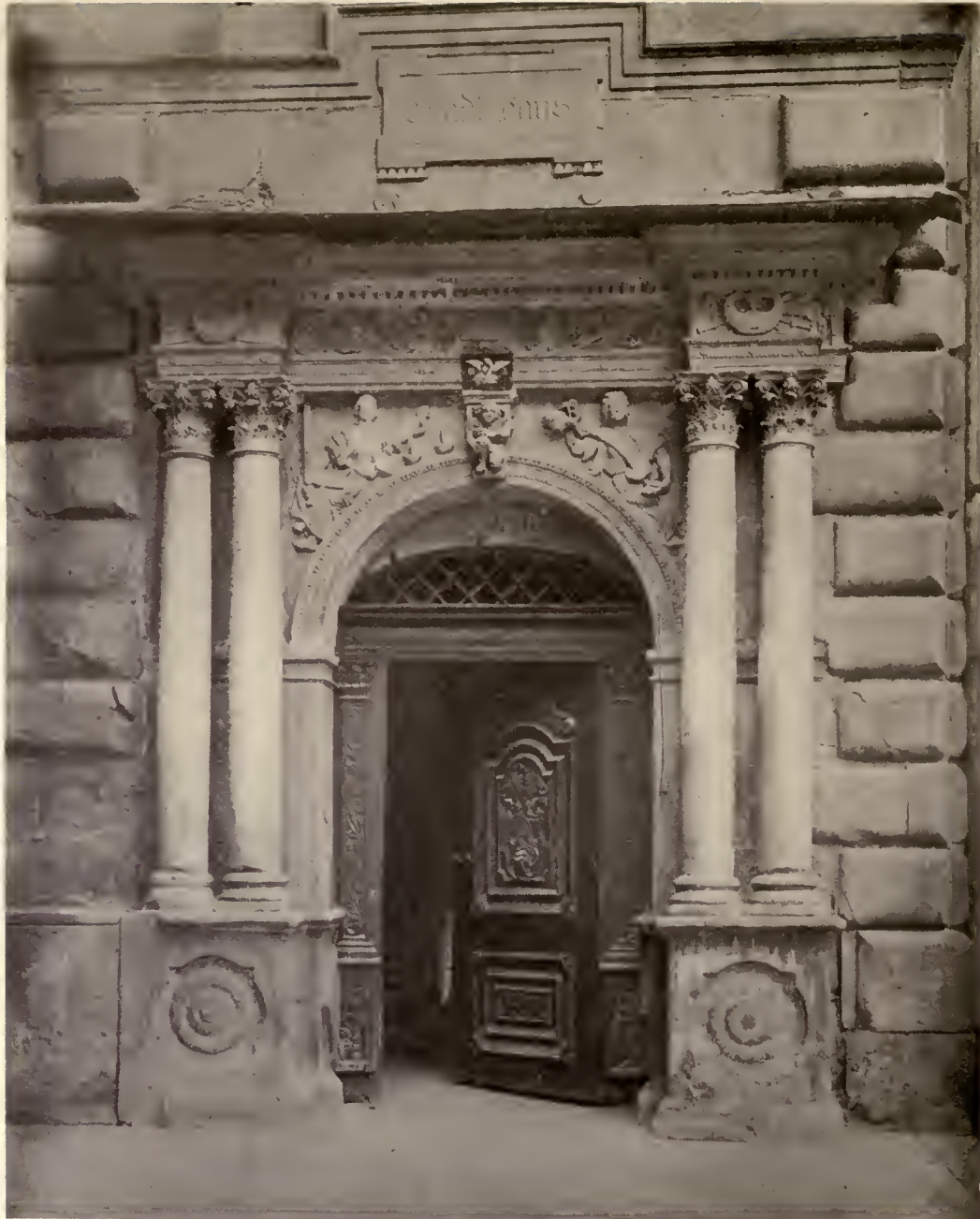
DETAIL OF DOORWAY—RATHAUS, LUCERNE
